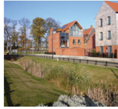
Drainage features could be a key feature of new development
