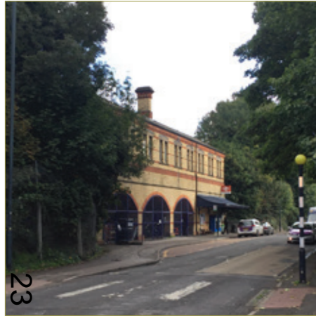
Maidenhead Railway Station access off Shoppenhangers Road
